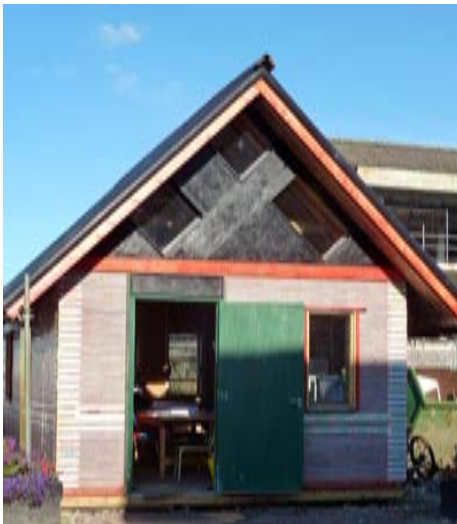
The new visitor centre, made out of reclaimed materials. Photo by Neil Clarke
